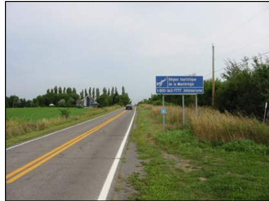
Route 225 (Quebec) looking north. Much of this 2-lane road is only 16 feet wide.
