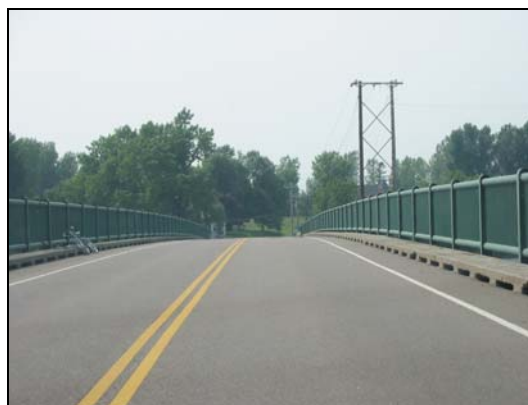
Route 2 bridge linking North Hero and Alburg (looking west)
