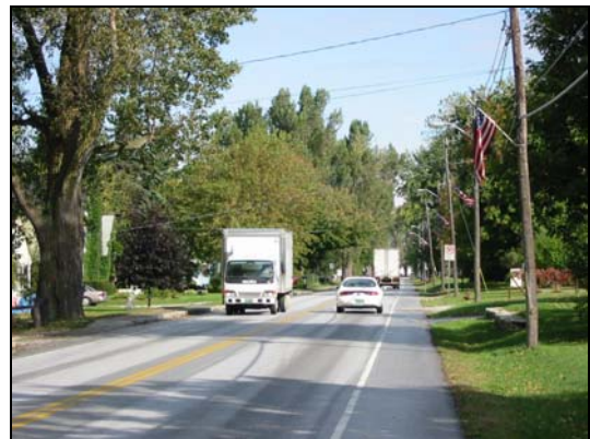
Route 2 (Alburg) north of West Shore Rd looking north. This 2-lane road is 30 ft wide with 11 ft lanes and 4 ft shoulders.
