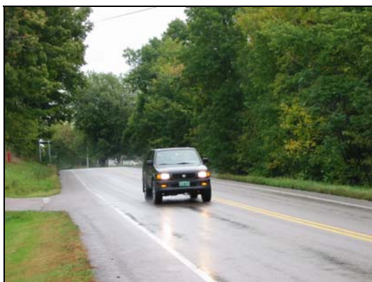
Route 2 at North Hero Elementary School looking north. This 2-lane road is 30 feet wide. Travel lanes are 11 ft wide with 4-foot shoulders.
